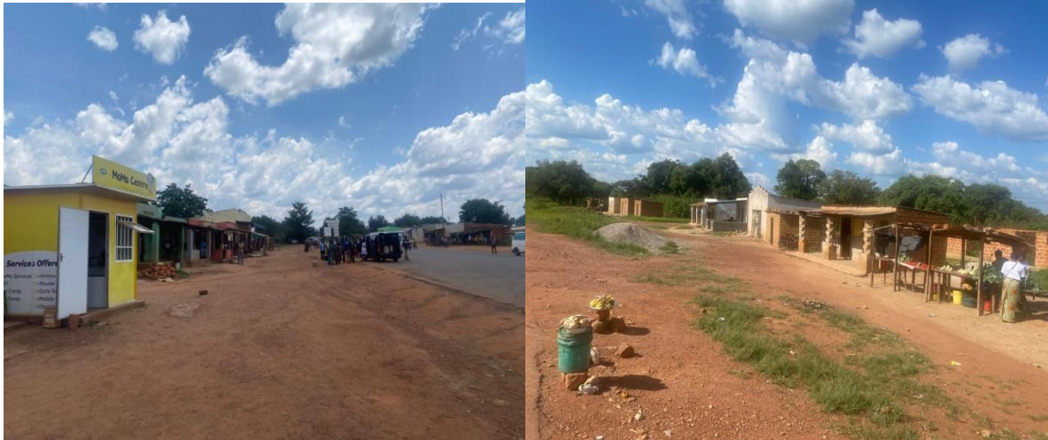
Figure 27 Typical Infrastructure on the side of existing road.
